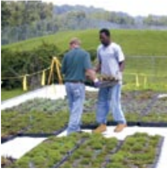
Top: Each two-foot-square plastic flat is placed directly on top of geotextile felt pads.
